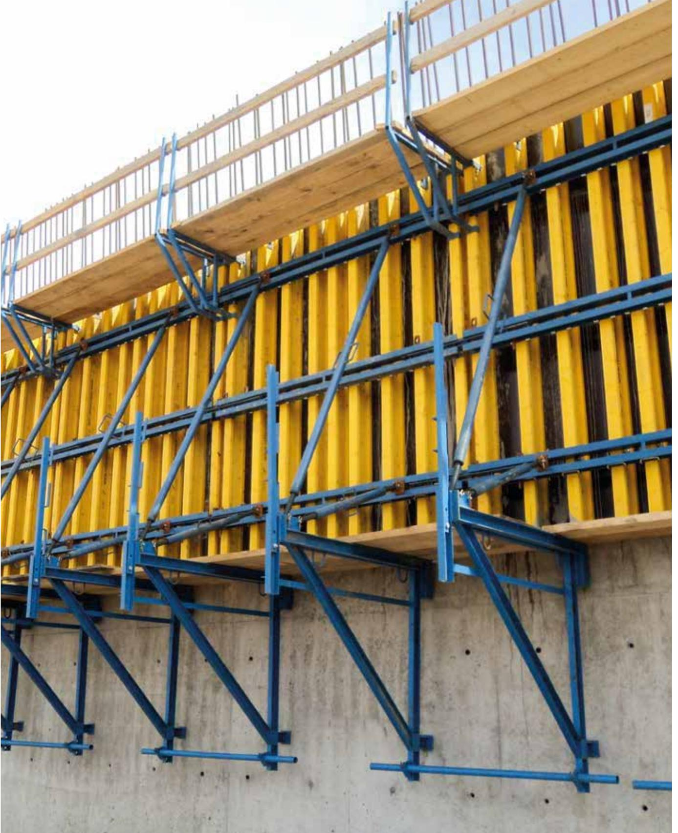
Climbing systems are used for walls and columns. Climbing consoles are fixed to the concrete by means of climbing brackets or conic anchors. By creating a platform on the consoles, the surface on which the wall and column formwork will sit is obtained. In addition, a safe working area is created for the workers.
