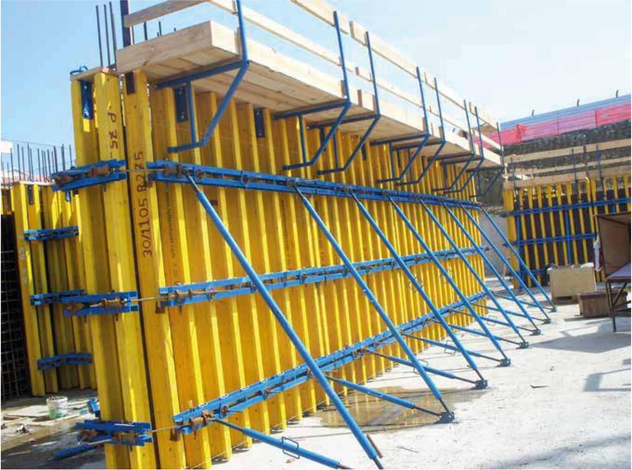
By using H20-H20 belt joining component, different heights can be obtained and it gives the opportunity to use H20 wooden beams as a single beam.
