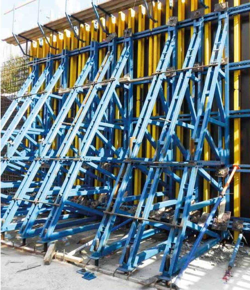
Single-sided formwork systems are used in cases where the wall formwork cannot be mutually connected, and anchorage shafts cannot be used.
